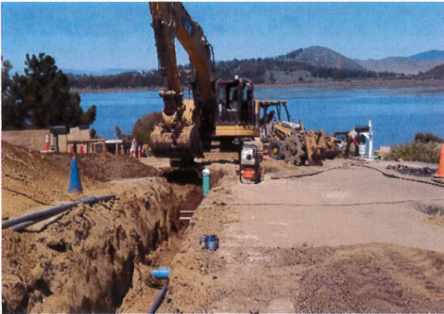
Figure ES-3. Los Osos Wastewater Project Pipe Installation (2013)
